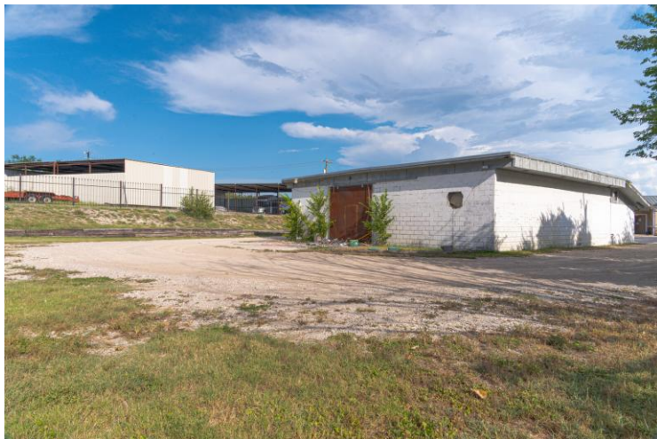
Office structure — site fronts the active US-377 growth corridor
