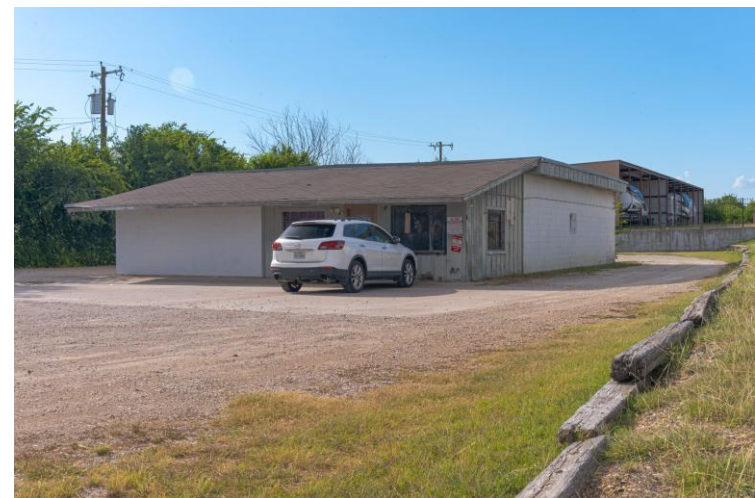
Storage building with additional metal warehouse structures beyond
