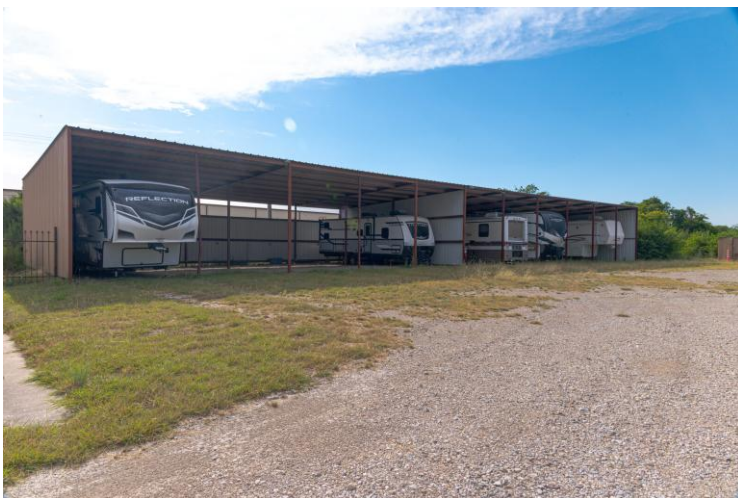
Concrete block storage building
