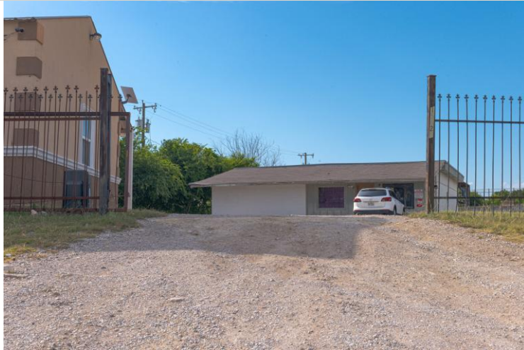
Office / residence structure near the site entrance
