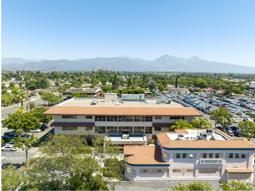
North facing view
