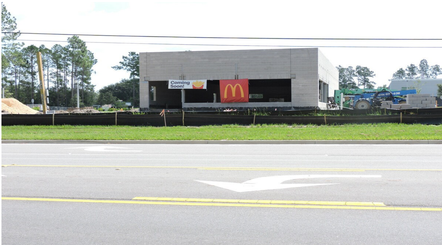
McDonalds Under Const Across St
