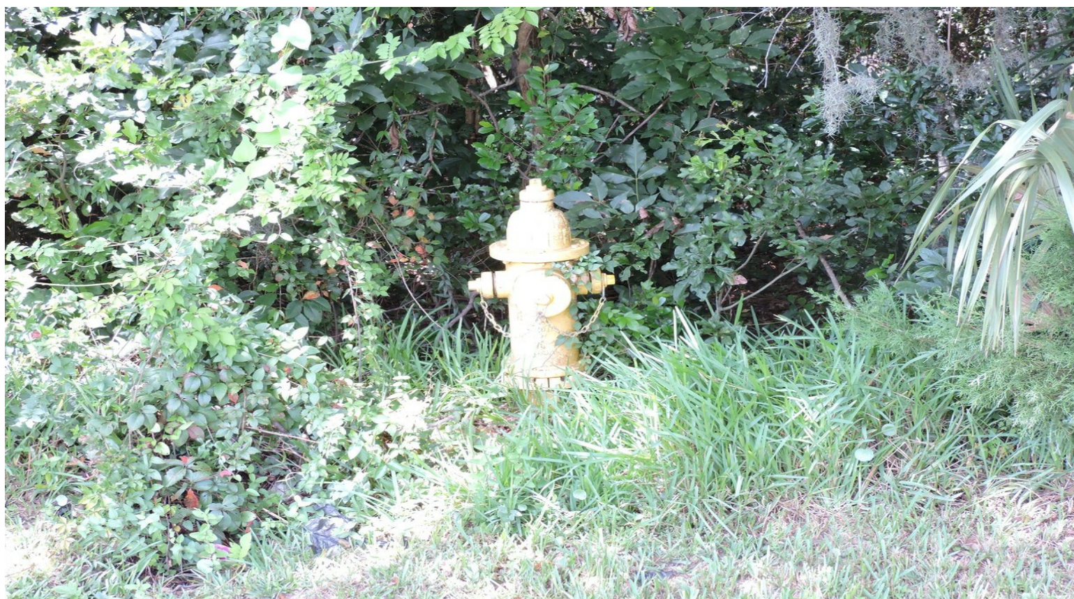
Water at Site
