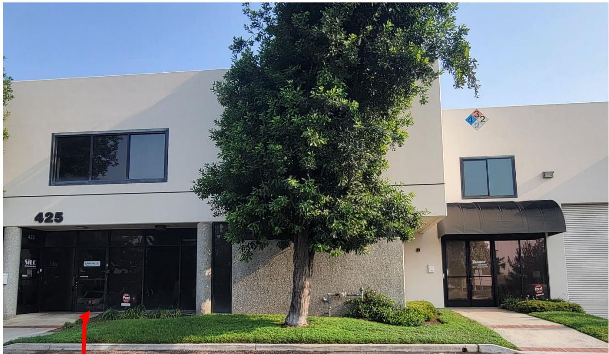
Entrance to 5,000 sq. ft. Lab/Office Space
