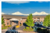
MedLine ReNewal Headquarters in Redmond.
