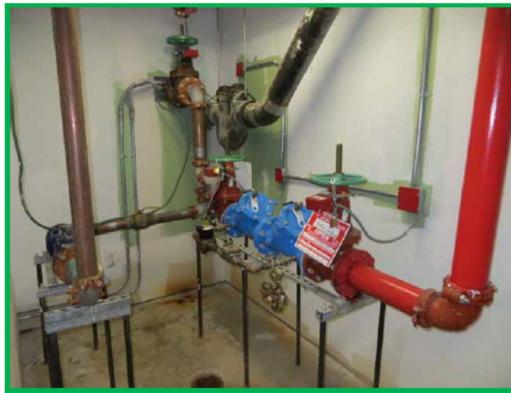
SPRINKLER CONTROL VALVES
