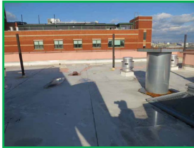
VIEW OF THE ROOF
