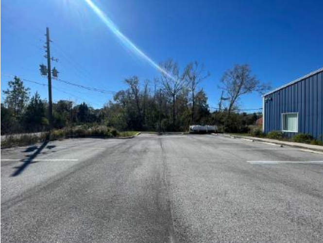
43. Pole Mounted Transformers
