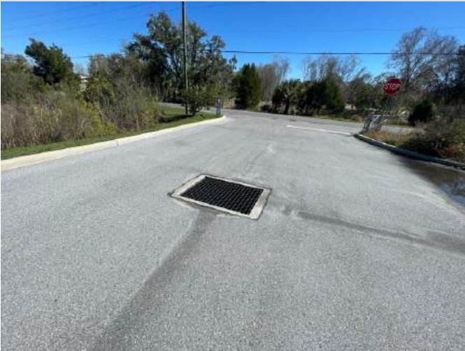
45. Stormwater Drain
