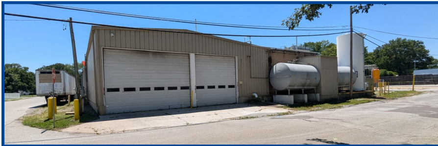
Back of Building facing W. 5th Street
