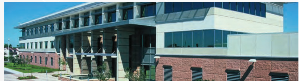
FBI Facility | McAllen, TX ( \pm 80,000 SF)
