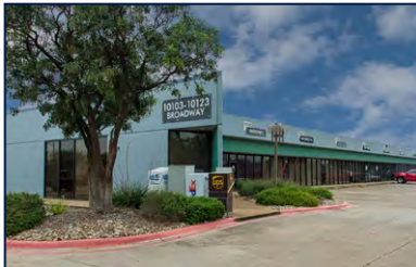
Bldg A 9921 - 9929 Broadway
