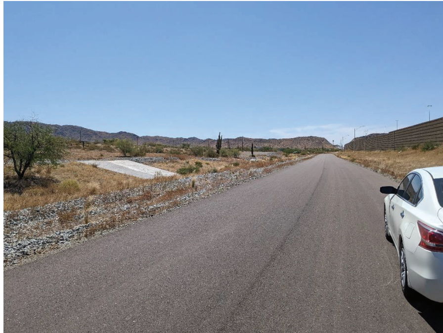
Site looking E-along Dusty Ln (202 right behind wall) (172011088)
