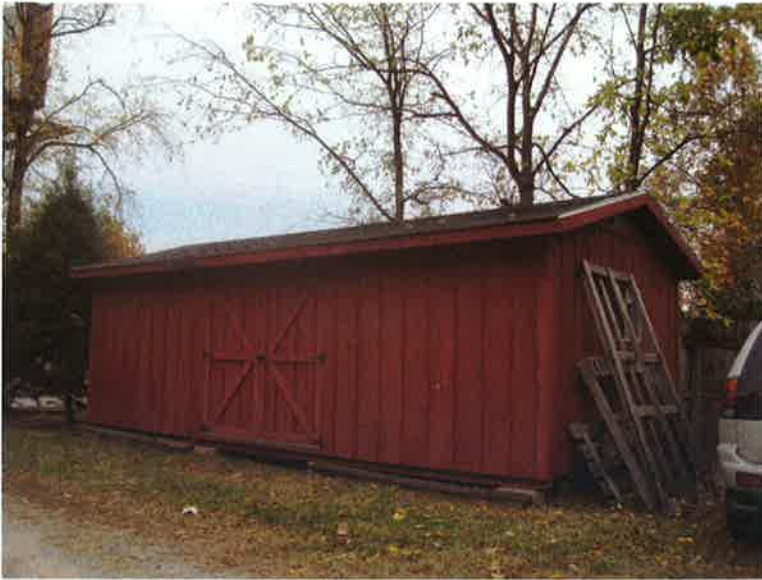
Storage building on the subject property.
