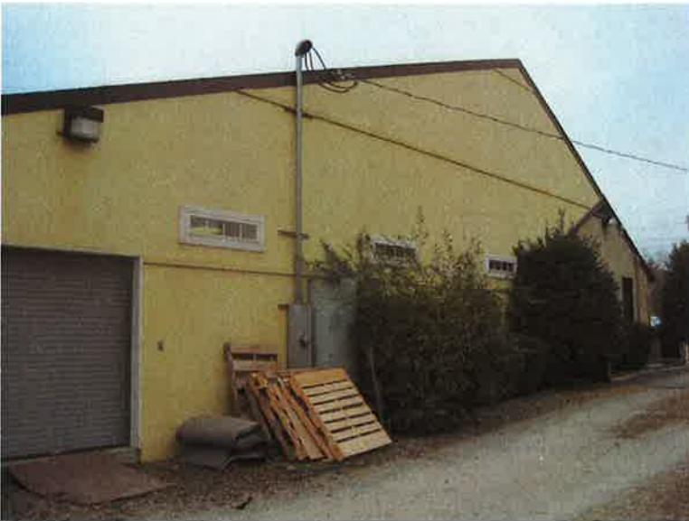
North wall of the subject building.
