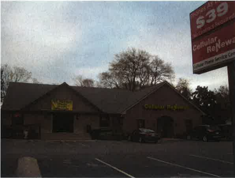
Front view of the subject building.
