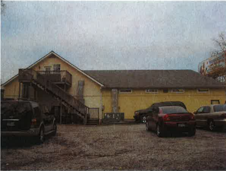
Rear view of the subject building.
