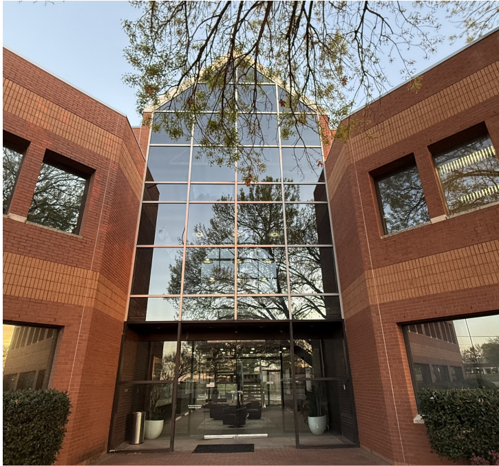
Atrium Front Entrance
