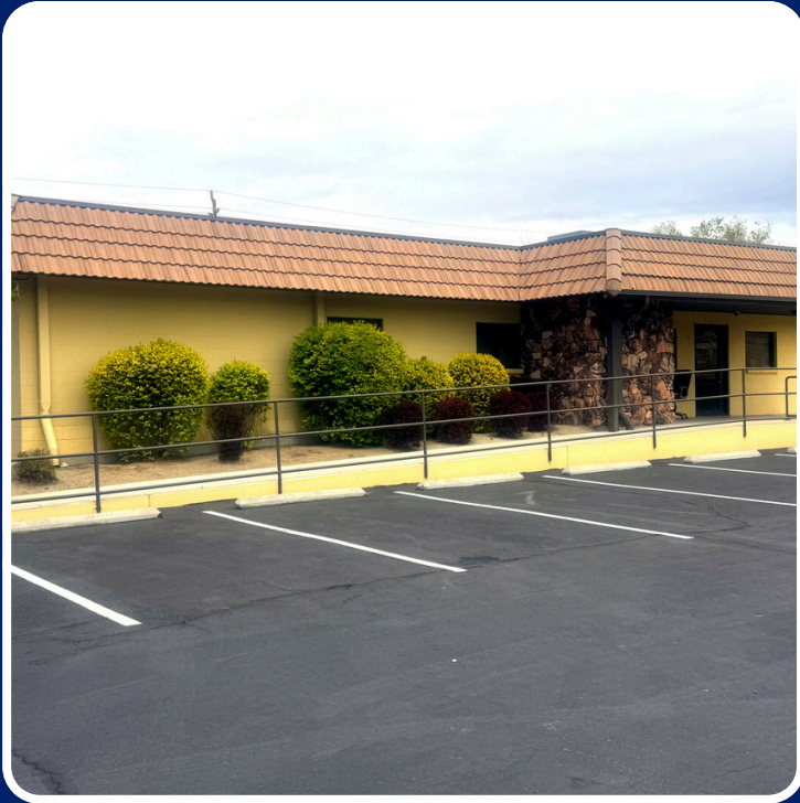
REAR OF BUILDING
