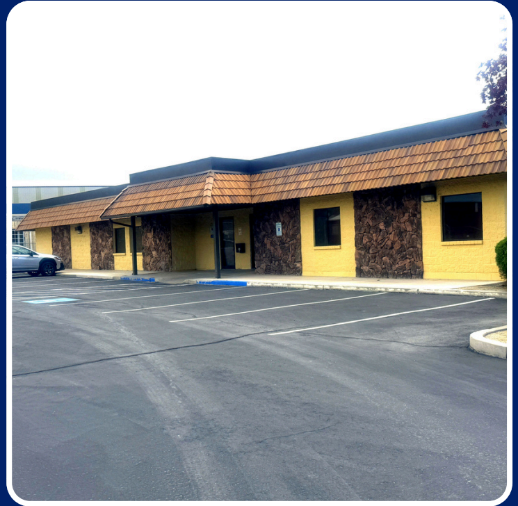
FRONT OF BUILDING
