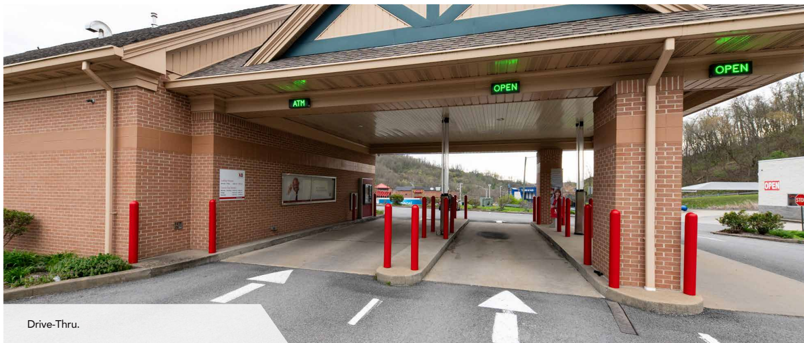
Exterior Back of Building.
