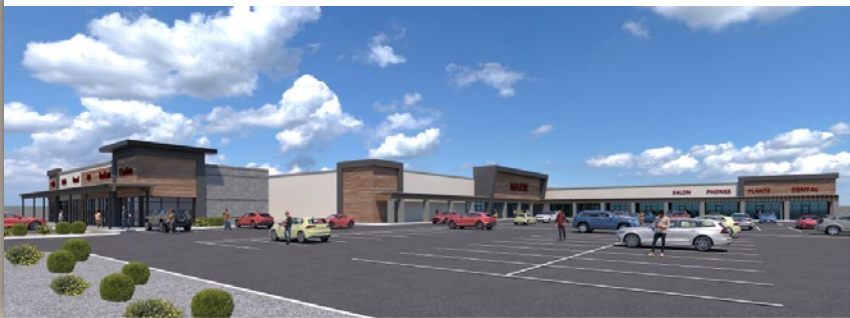
Excobedo Plaza (Renovation Under Construction)
