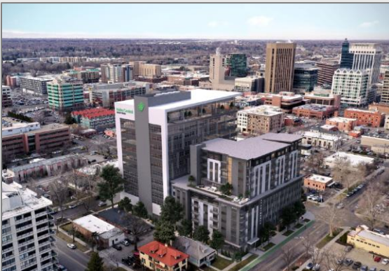
ICCU tower, 125 apartments, ~170,000sf of office & retail Photo courtesy of Design Review
