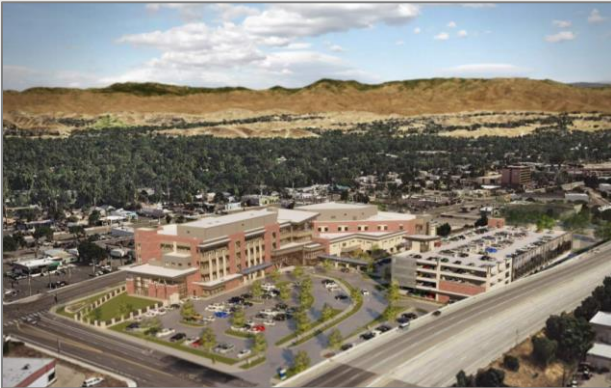
St. Luke's, 230,000sf orthopedic hospital, ~600 space garage Photo Courtesy of Design Review
