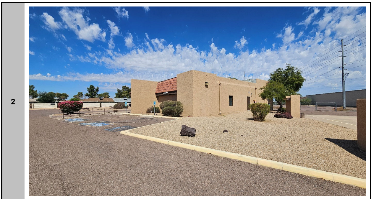
View northwest toward the subject building
