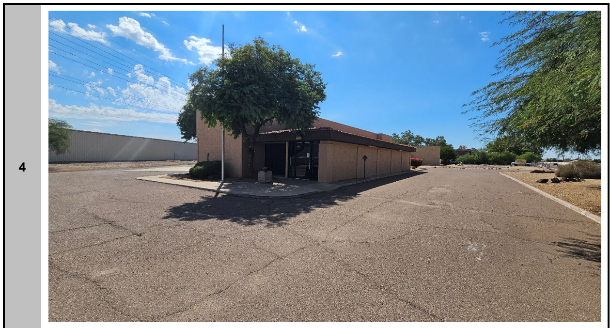
View southeast toward the subject building
