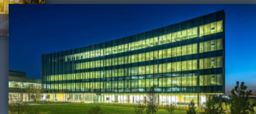
Anadarko Petroleum Building
