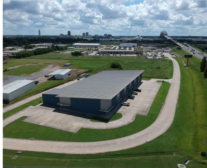
View from West to East
