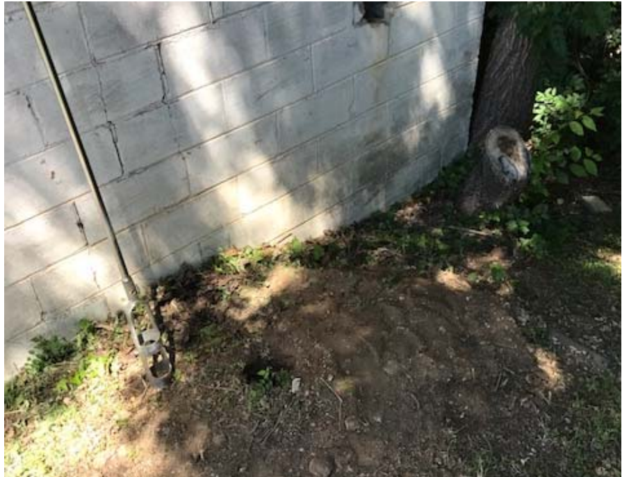
Photo 3: View of hand auger soil boring B-5 located on the eastern exterior wall of the garage.
