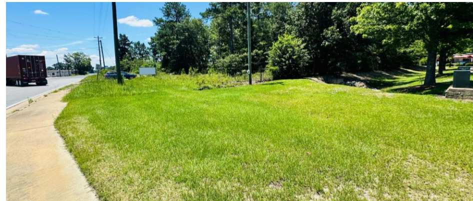
Sidewalk Along Firetower Road
