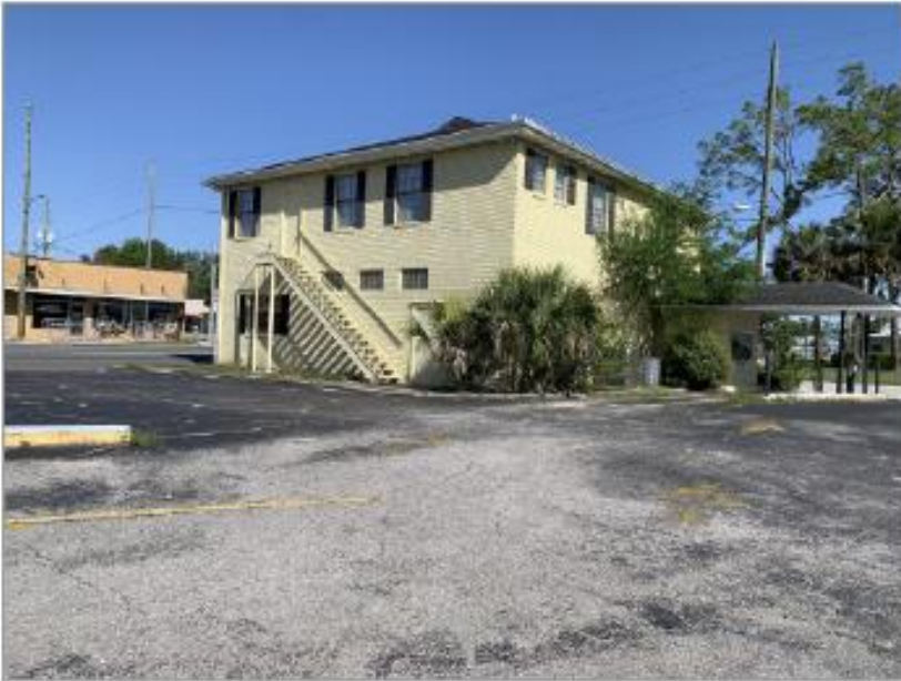
Southern side of subject building
