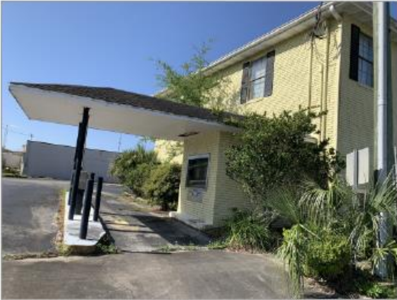
Eastern side of subject building with drive-through lane
