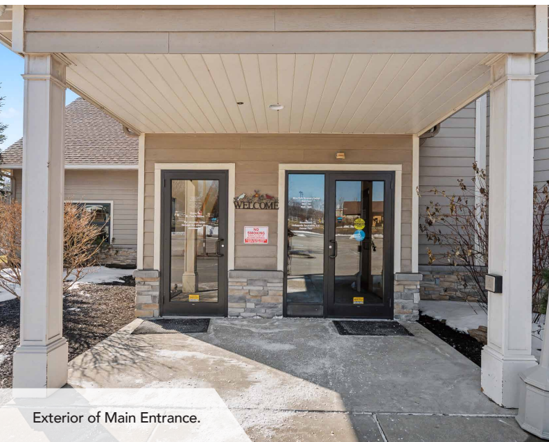
Exterior of Building.
