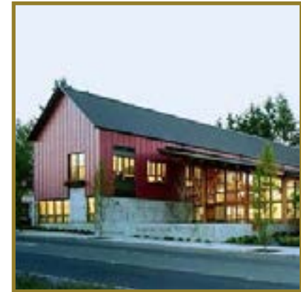
Small Retail Building
