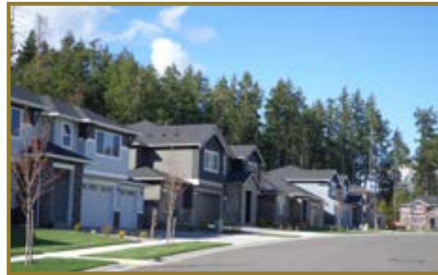
Streetscape / Varied Rooflines
