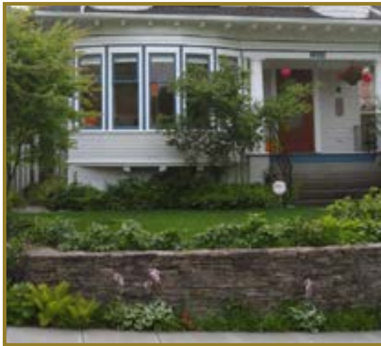
Front Yard Retaining Wall
