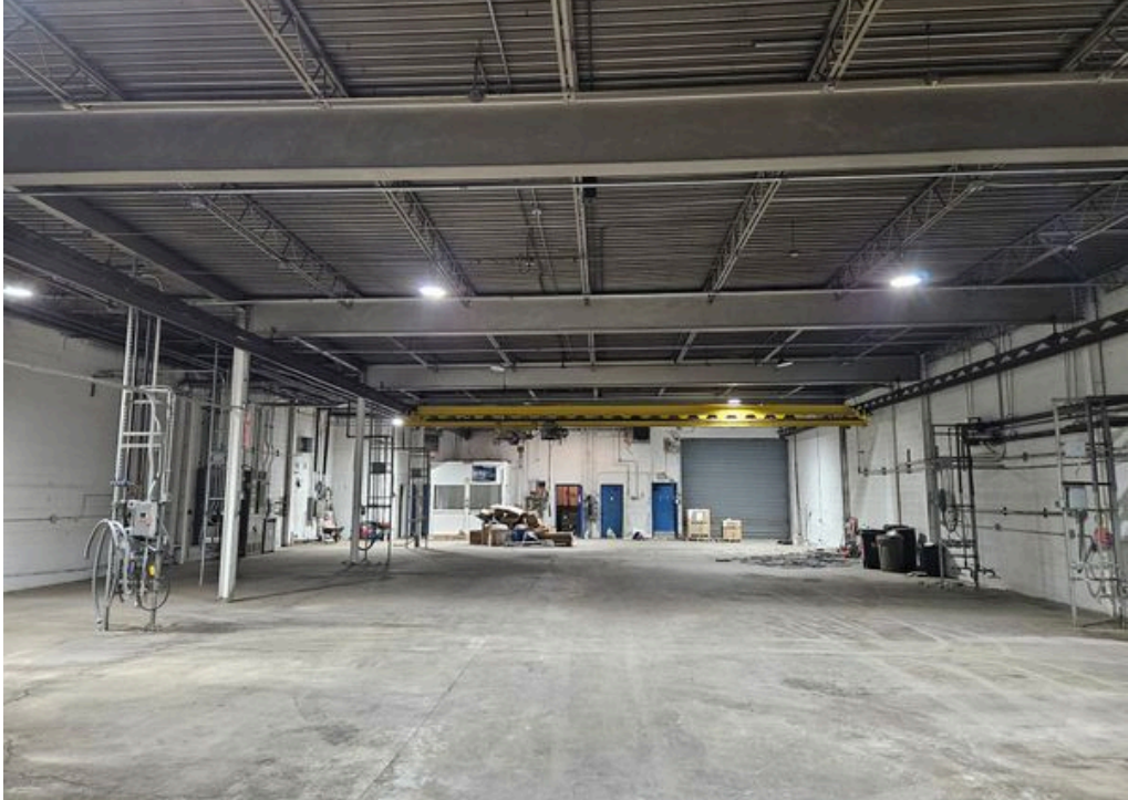
Shop with Crane
