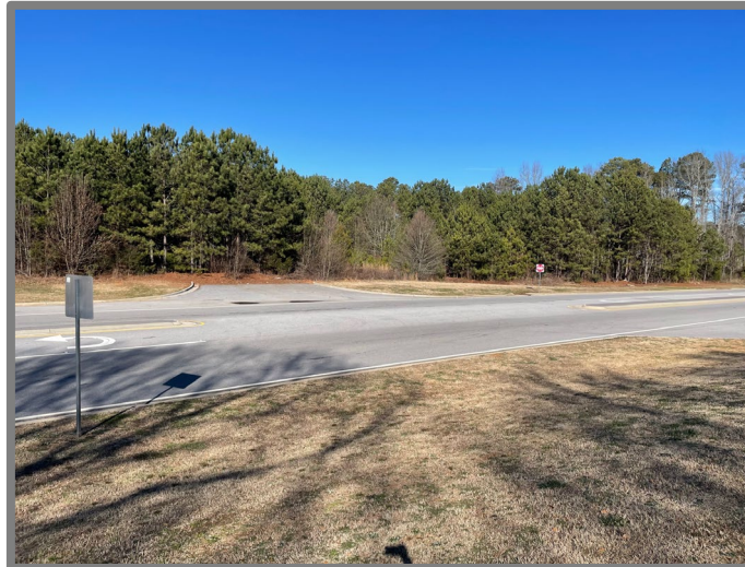
Existing Median Break
