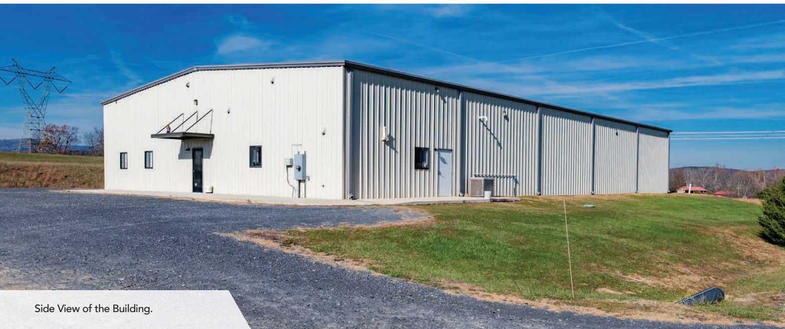
View of the Main Entrances.
