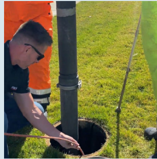
Vacuum removal of debris
