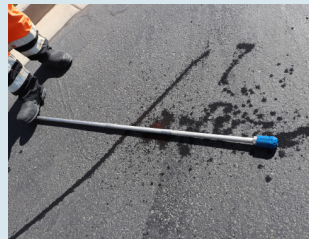
Wand used to loosen debris
