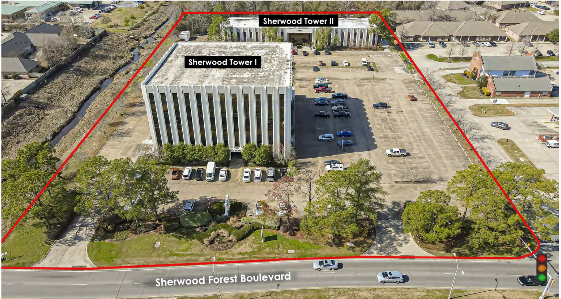
Sherwood Towers I and II (Additional Square Footage Also Available in Tower II)
