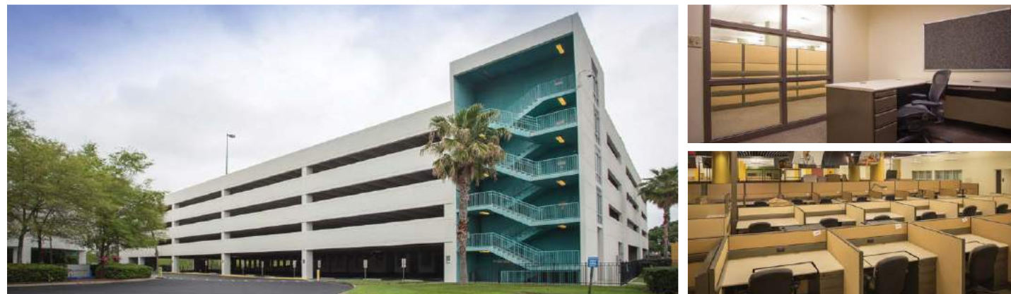
Private garage, private office, and workstations.
