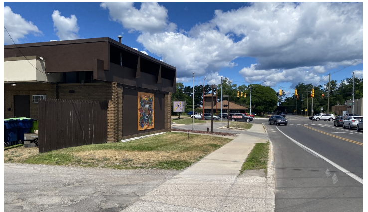
SE Corner Looking North
