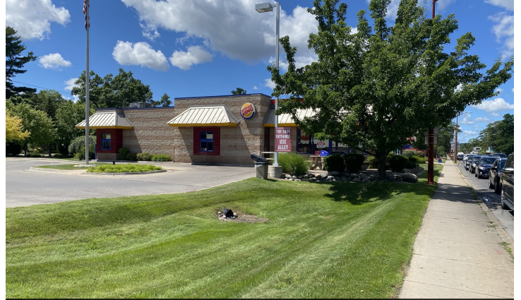
SE Corner Looking West
