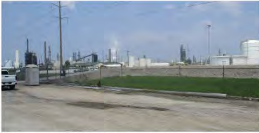
Coffeyville Resources Refinery (10 miles from the park)
