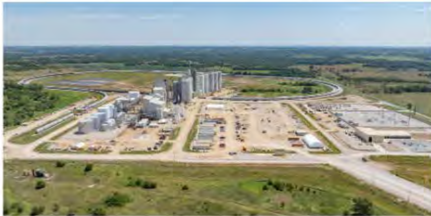
Bartlett Soybean Crushing Plant (10 miles north of the park on Hwy I69)
