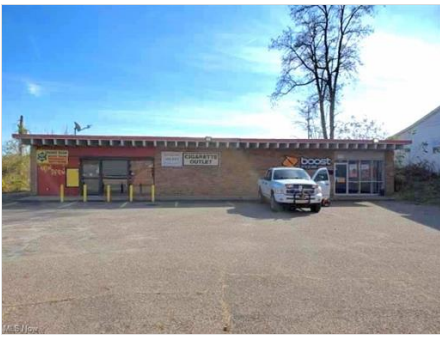
Front of Structure
