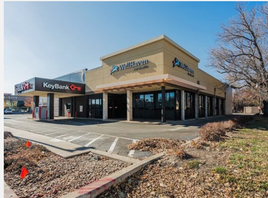
2305 S Colorado Blvd, Denver, CO
