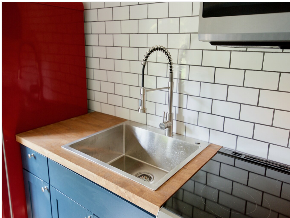
3rd Floor - Kitchen Detail
