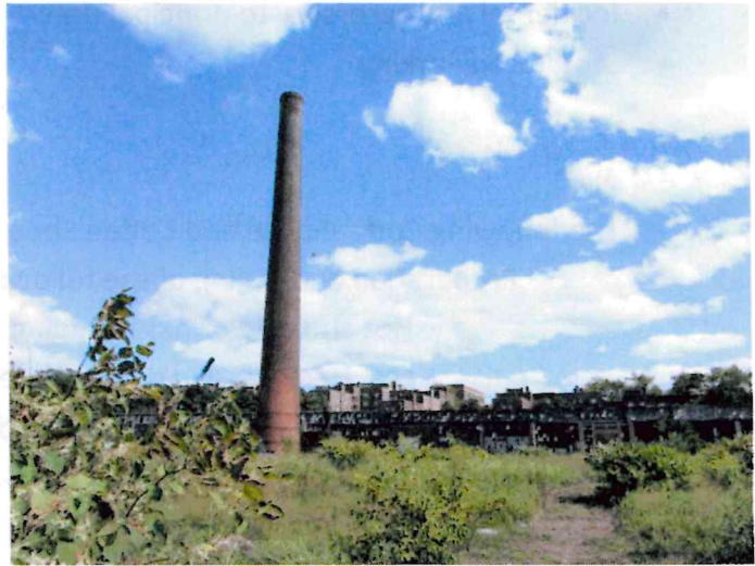
Airlite Aluminum Corporation Bat Factory Abandoned after May 27, 1986 Explosion
