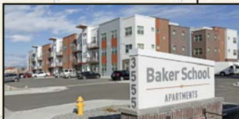
BAKER SCHOOL APTS. 3555 W 64TH AVE. BUILT 2019 / 142 UNITS
