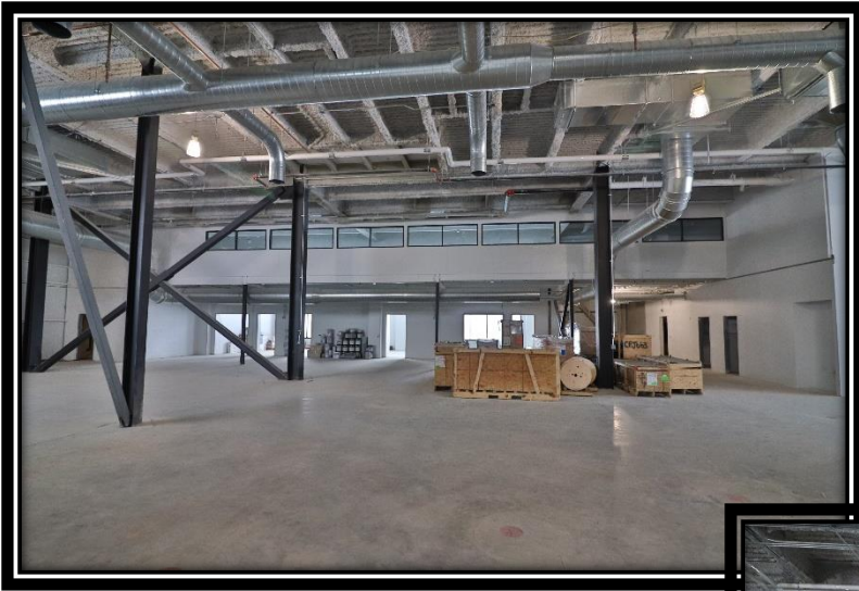
1 st Floor- Looking at Office
