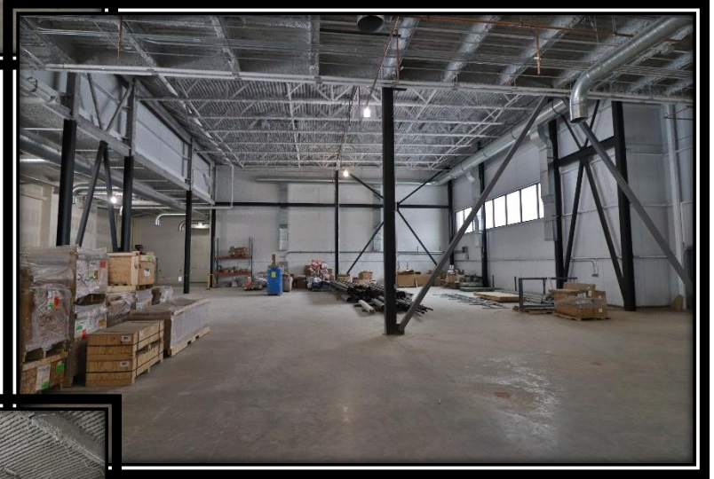
1 st Floor- Looking West
