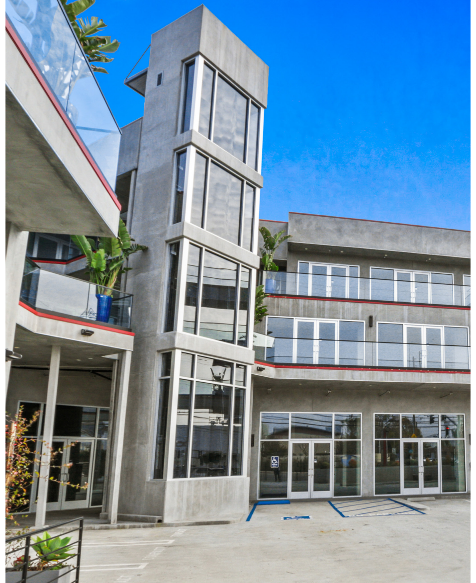
Elevator access to all floors
