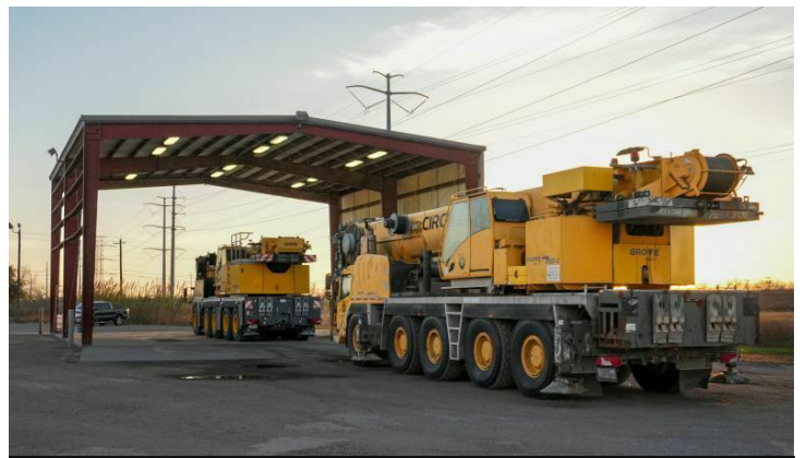
2,750 SF Wash Bay
