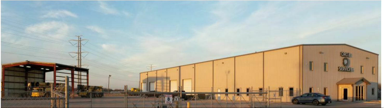
The wash bay and expansive stabilized limestone yard make this site ideal for fleet operations, equipment staging and outside storage.
