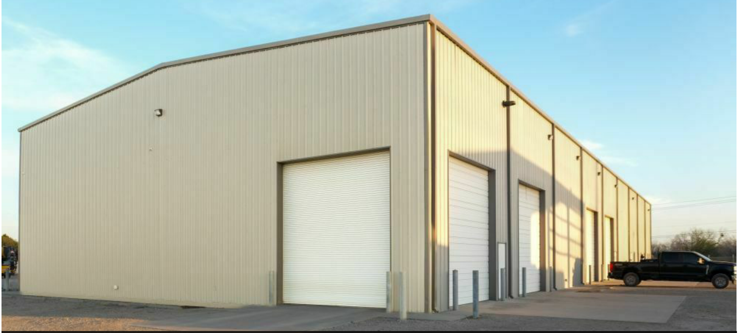
Four (4) overhead doors are located on the west side, and one (1) is located at the rear of the building.
