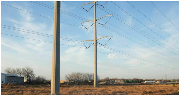
The property is traversed by one (1) 345-kilovolt (kV) & one (1) 100-161-kilovolt (kV) U.S. electric power transmission lines.
