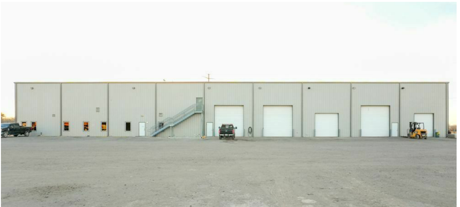
Five (5) overhead doors are located on the east side of the building.
