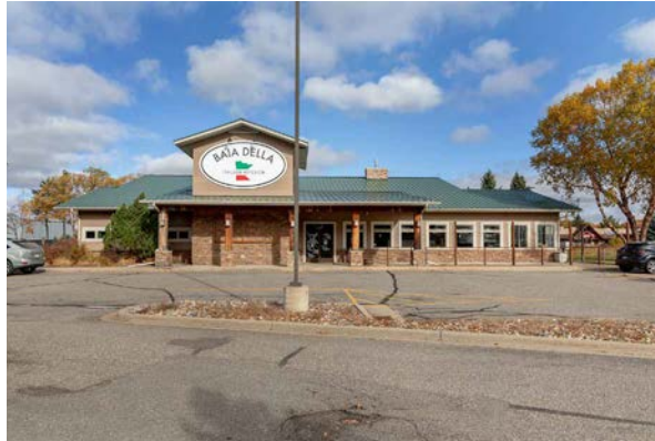
Front of Building
