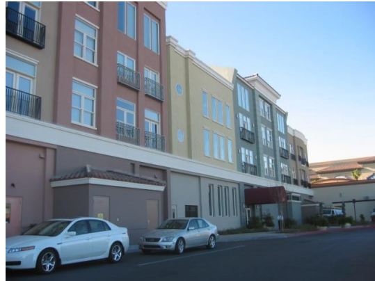
Figure 1228-C: This figure shows two methods of using architectural features to create wall surface relief on wall elevations that are not the primary elevation.
