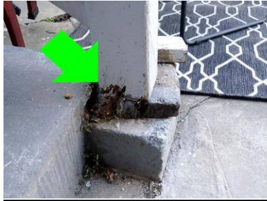
Post damaged and cut joist
