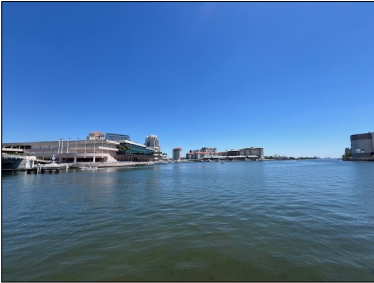
East elevation View
