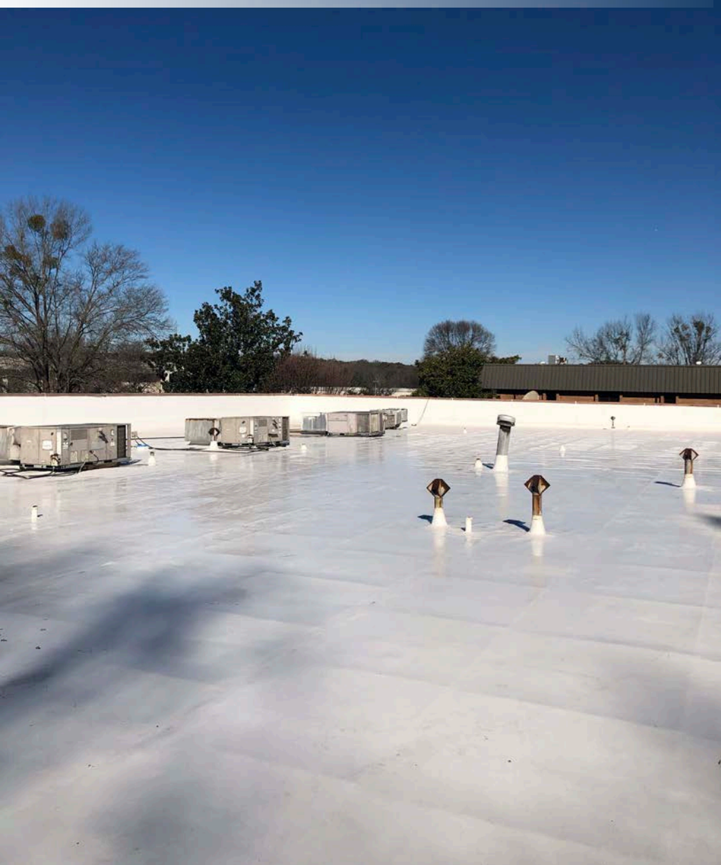
New TPO roof installed 2024
