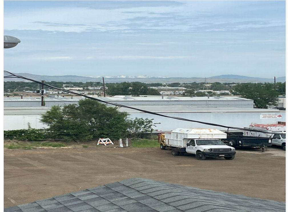
Roof Santa Fe looking West 1
