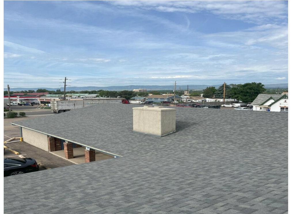
Santa Fe Roof looking South 4
