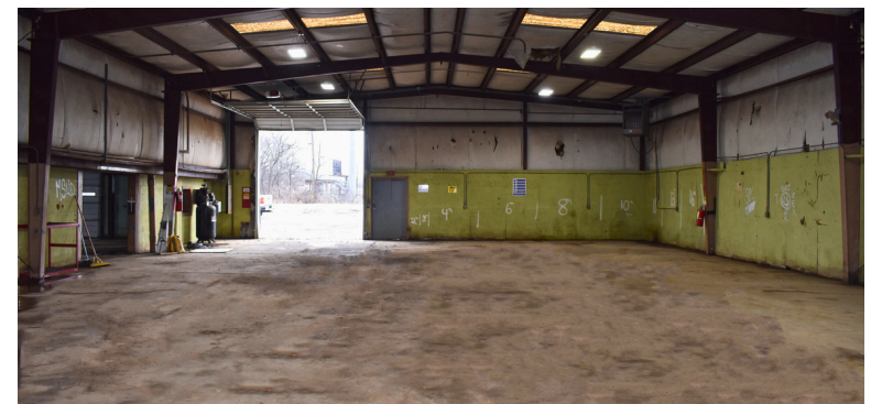
Clear Span in Half of Building
