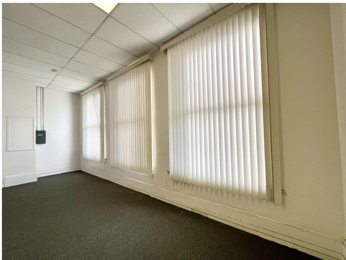
2nd level office space
