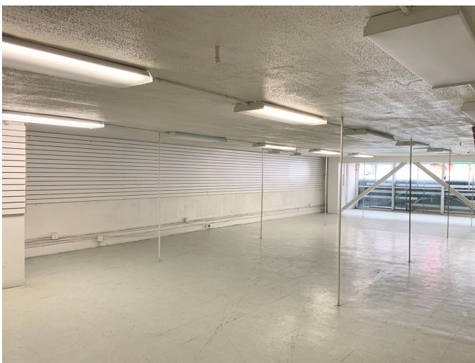
Mezzanine level storage
