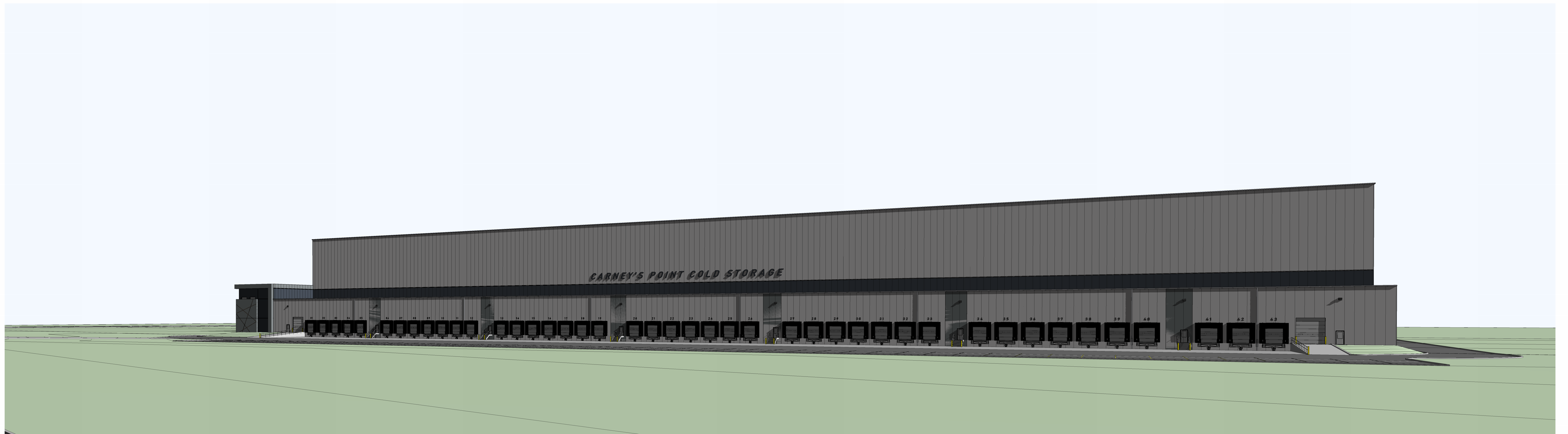
VIEW FROM HAWKS BRIDGE ROAD EAST
